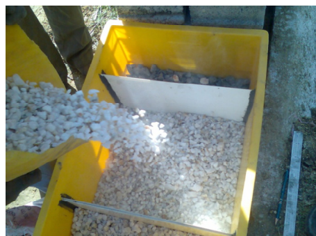
Fig. 2 Constructed wetland pilot unit PAPS
